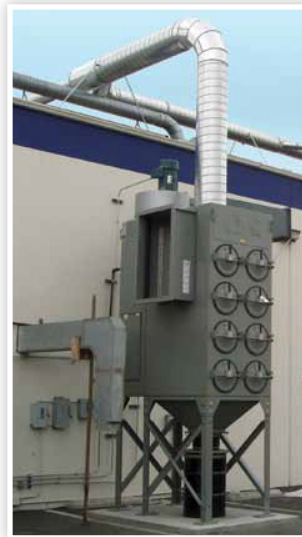
DustHog SFC 16-4 used for blending nutritional powders.
